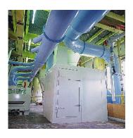
Acran acoustic enclosures are a modular design which utilise our acoustic panel system to provide a high level of noise reduction for both internal and external applications. Enclosures typically achieve acoustic performance between 15dB(A) and 25dB(A), with higher performance systems available.
